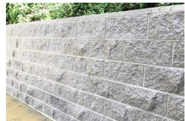
8 FOOT TALL 10 SPLIT FACED CMU WALL CALSTONE COLOR GREY 100 NOT TO SCALE
